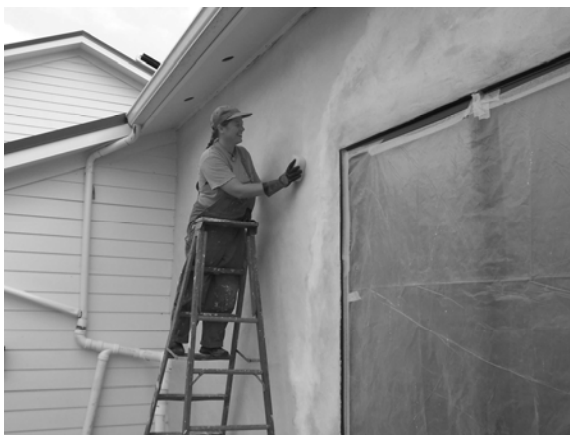
Mollie Curry applies lime plaster to SENS House strawbale wall.
