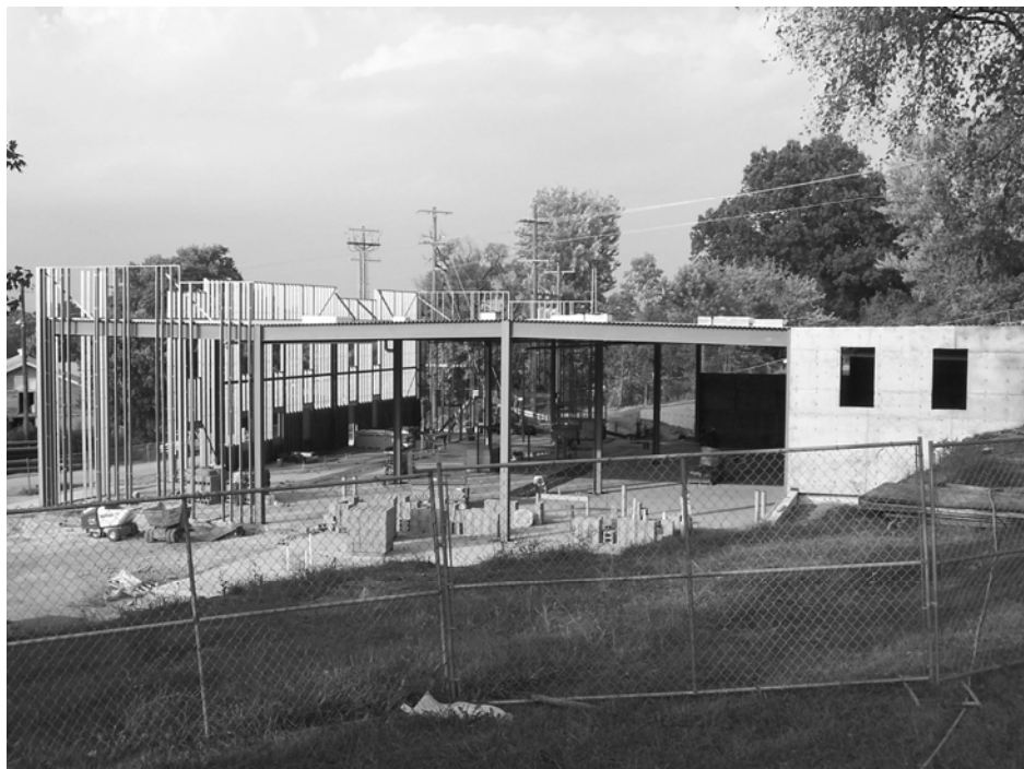
New Heat Plant in construction.
