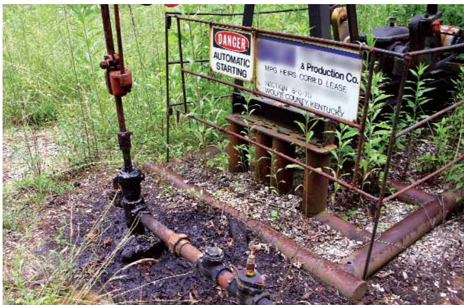
A leaking oil pump on the Sheltoewe Trace was recorded at GPS coordinates -83.7011484 and +37.7234965.
