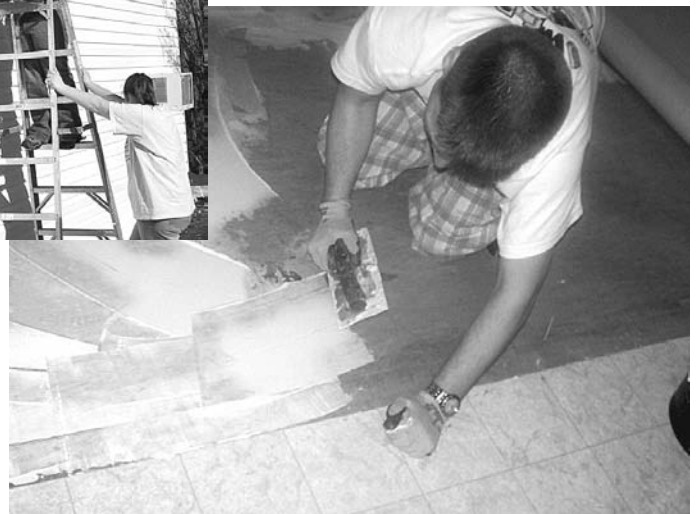
BELOW: Michael King, '09, glues flooring at the Charleston Habitat for Humanity Office.
