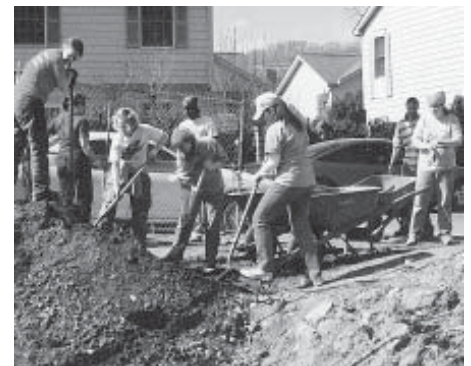
Berea College students work on site in New York City.
