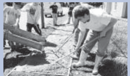
Habitat for Humanity members mix concrete during Spring break.
