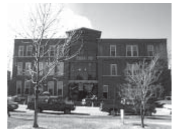
Bruce and Trades before (top) and after (above) renovation. The Connector joins the two buildings.
