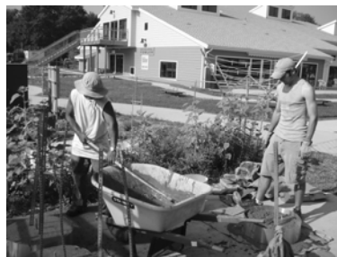
Students mix concrete for shed footings.
